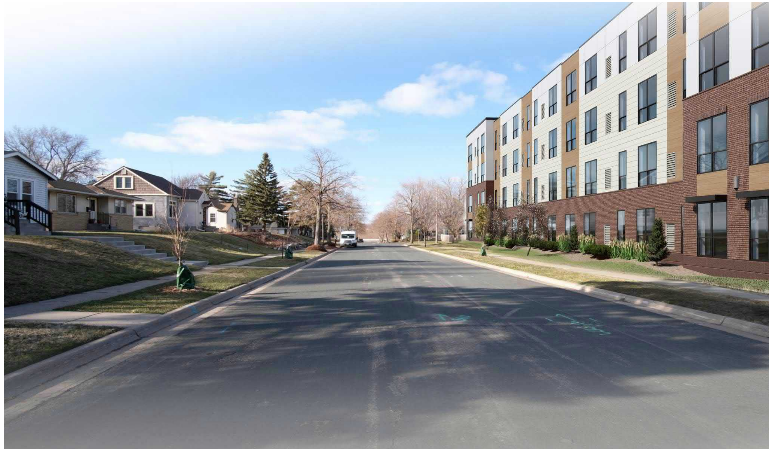
VIEW NORTH ON JACKSON ST NE
